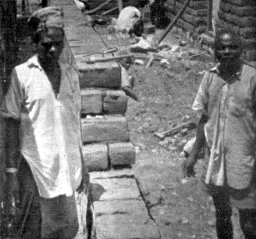
Rebuilding with sun-dried mud bricks.
