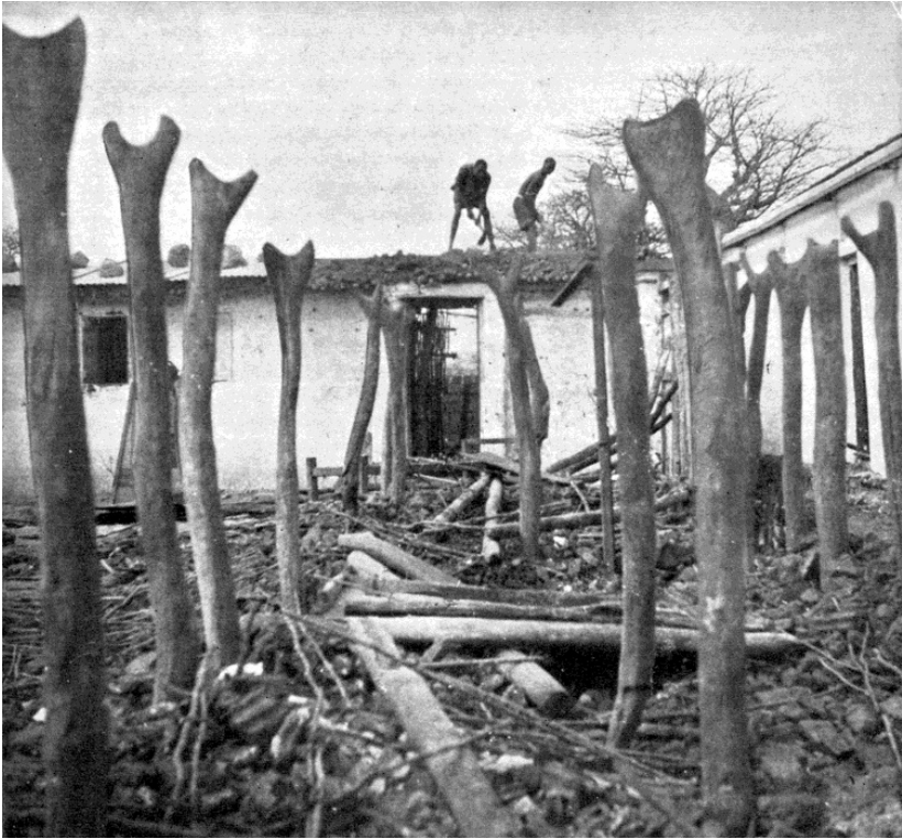
Pulling down the old men's ward, Mvumi Hospital.
