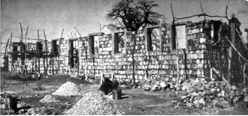
Building the new maternity ward, Mvumi Hospital.
